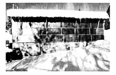
'The side and back walls were constructed using salvaged, cast glass, door fronts from old Herman Miller casework, with occasional cedar lattice inserts. The glass and cedar panels are wrapped around the supporting building volume like a large blanket suspended a distance from the tar paper underneath, forming an air pocket that heats up during the day and helps keep the building warm at night. The cedar was used for visual
